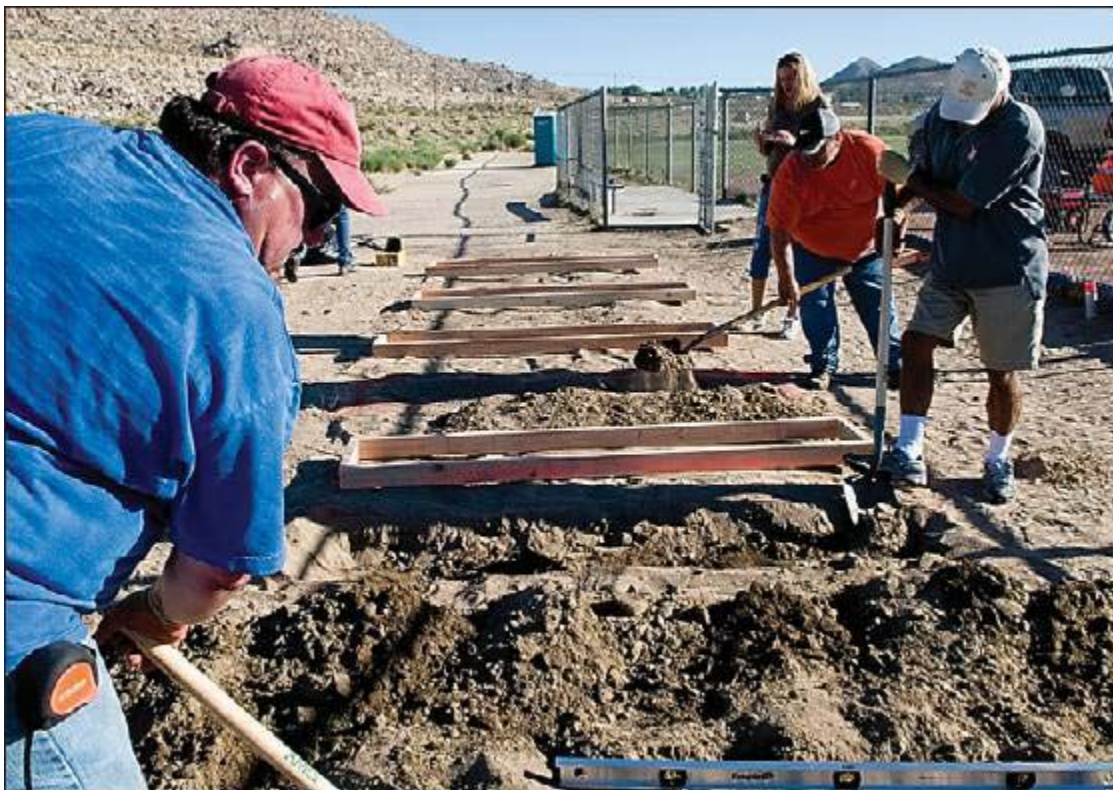
JAMES QUIGG, DAILY PRESS LAYING A FOUNDATION: Tom Neavill, left, places concrete forms for bleacher foundations at the Academy for Academic Excellence's softball field.
